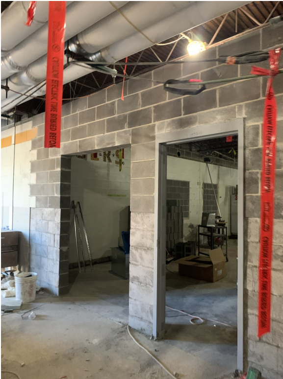
Area B East—New CMU Door and Window Opening
