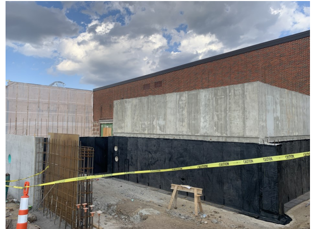
Area G—Addition 2 South—Foundation Walls
