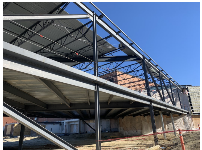
Zone C—Addition 2 North - Structural Steel
