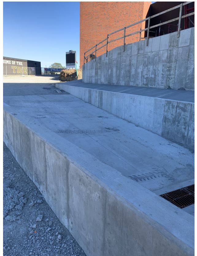
Loading dock for Deliveries
