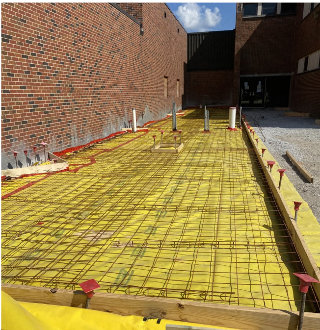
Addition—Slab on Grade Preparation
