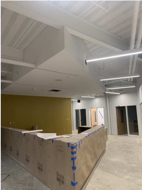
Addition—Level 1—Ceilings, lights and paint complete in open office
