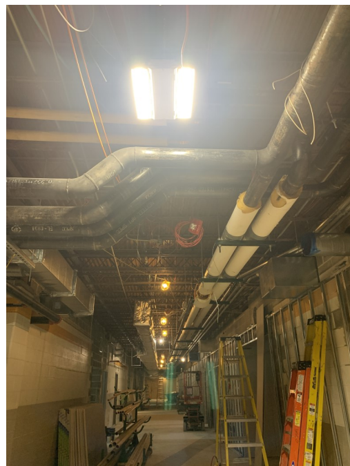
B Level 1 West—New overhead systems in hallway
