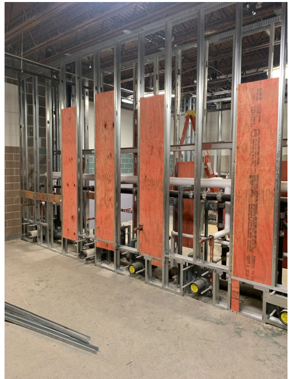
B Level 1 West—Restroom In Wall Plumbing and Fixture
