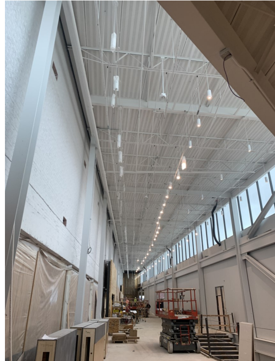
Addition— Pendant lights and freshly painted ceiling in clerestory
