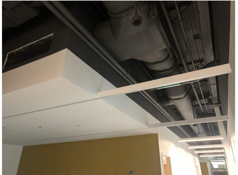
Addition—Level 2 - New linear light fixtures, ceilings, and painted
