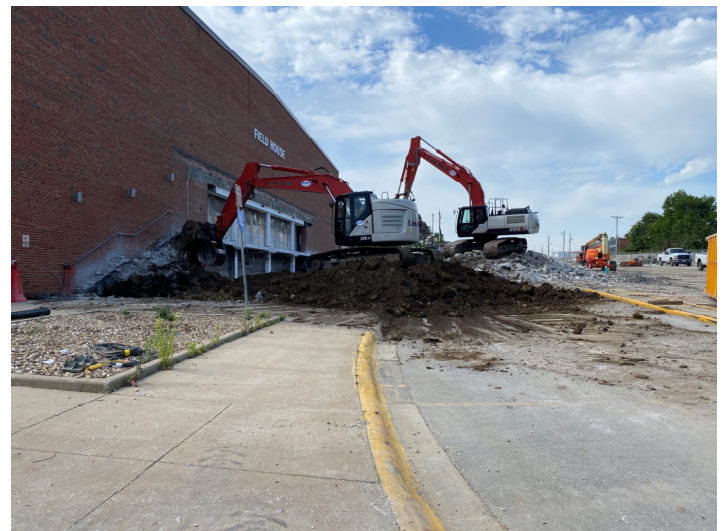
Area D & G Addition - Building Demolition
