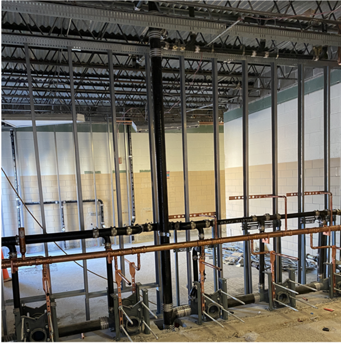
Area J - Level 2 - Bathroom Plumbing Carriers and Piping
