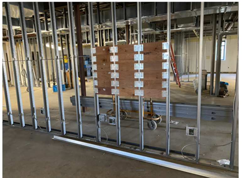
Area J - Level 3 - Electrical In-Wall and Backing for TV's
