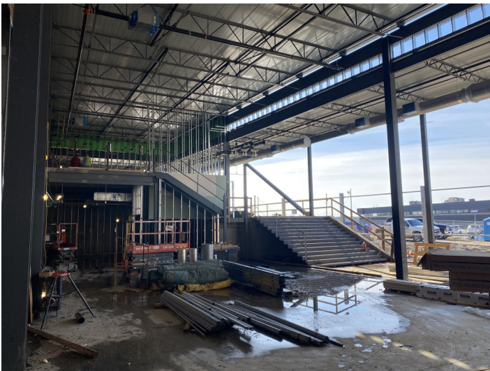
Zone G—South Addition 2 – Stud Framing and Roofing
