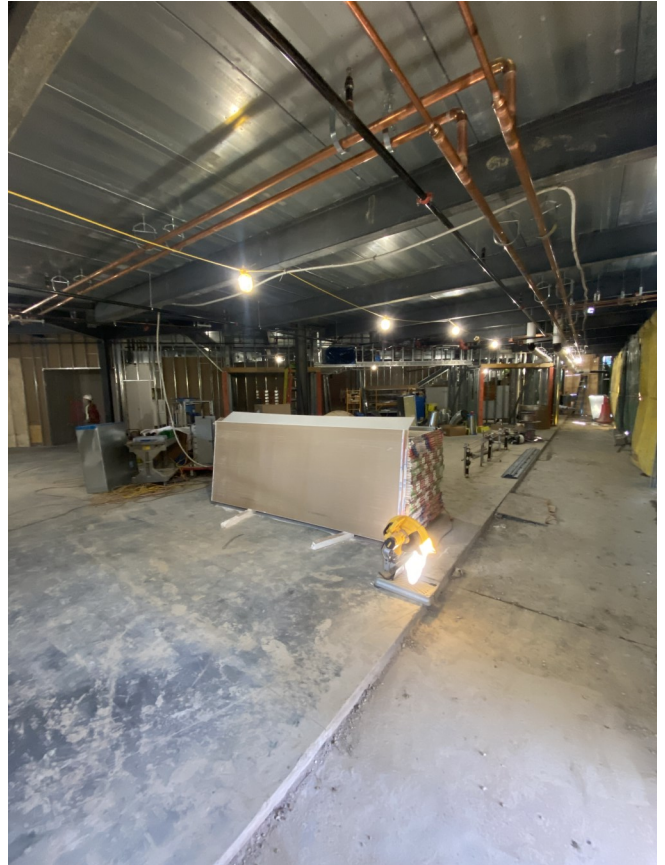
Zone C—Overhead MEP and Stud Framing
