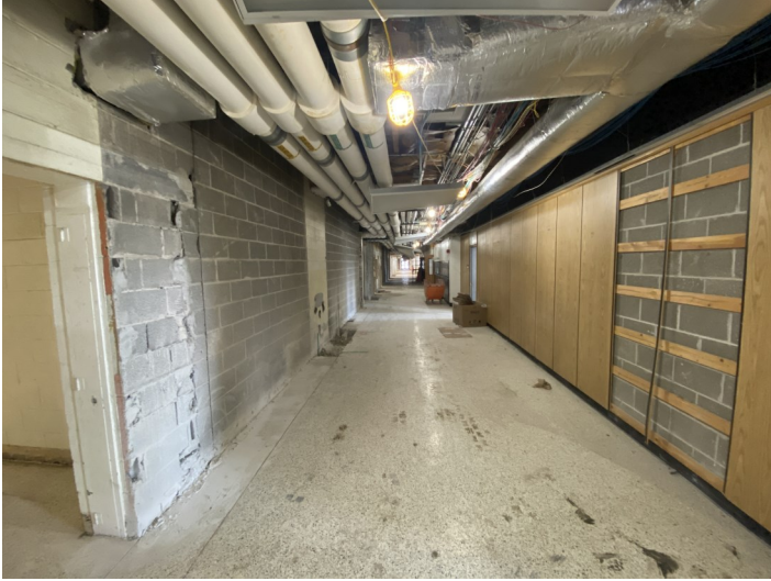
Zone K—Hallway Demolition
