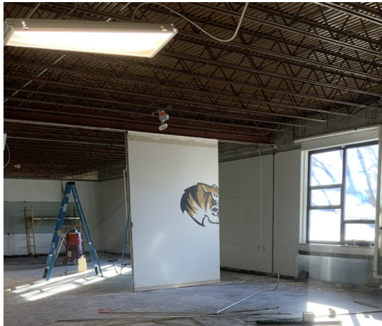
Addition— Level 2—Wood Wall Backup Framing and Overhead Sprinkler and Plumbing Systems
