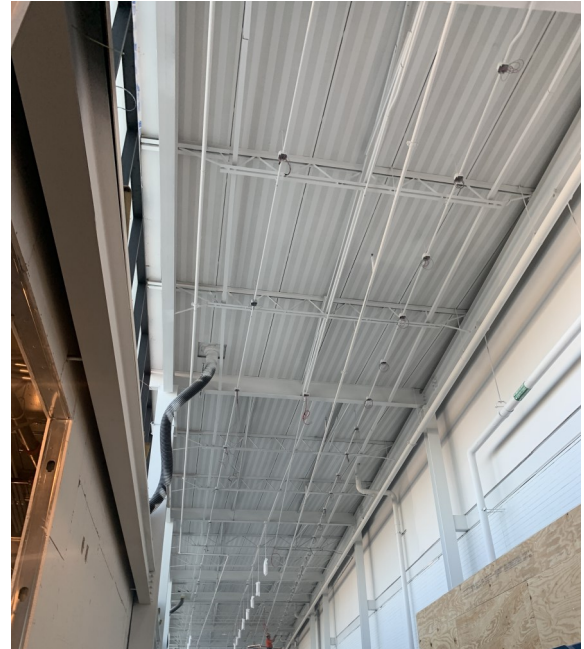
Addition— Pendant lights and freshly painted ceiling in “Innovation Way” Hallway
