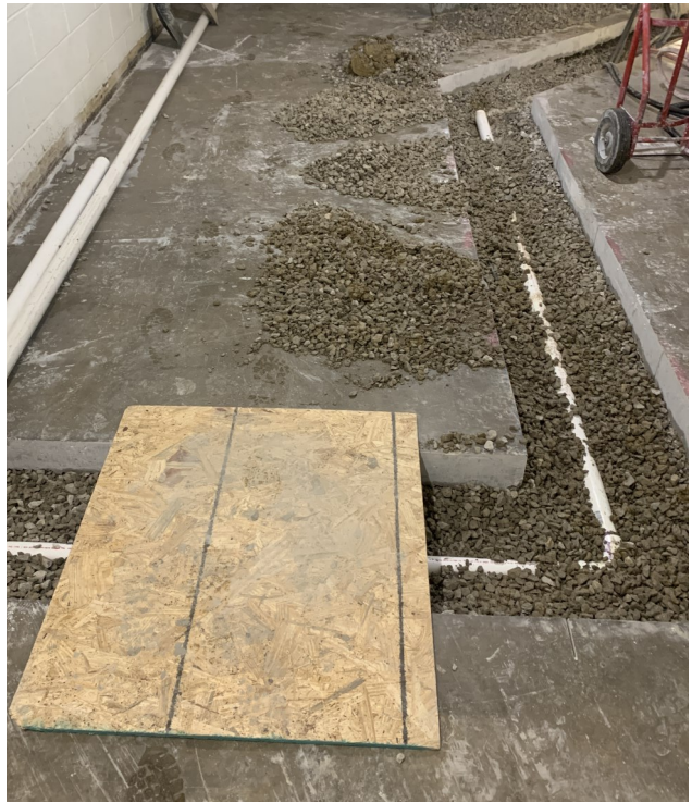
B Building Basement—Start of underground plumbing and trenching
