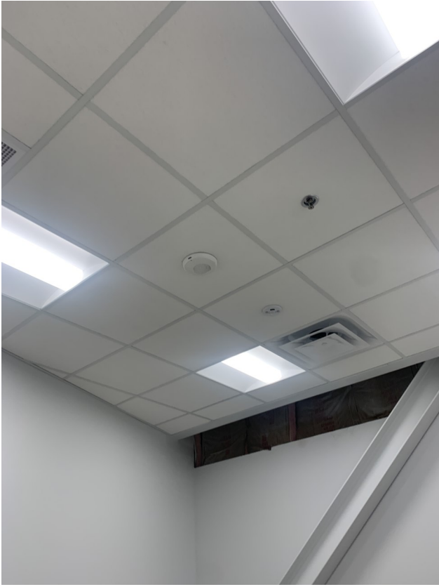
Addition—Level 1—Ceilings, lights and paint complete in offices
