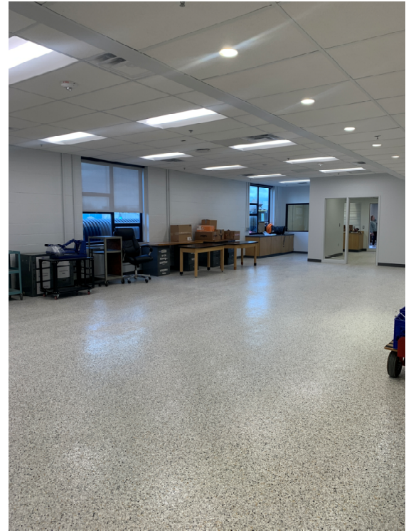
Zone B Classroom—Final Finishes
