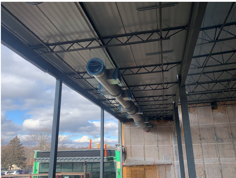
Zone G—South Addition 2 – Steel Complete and Overhead In Progress
