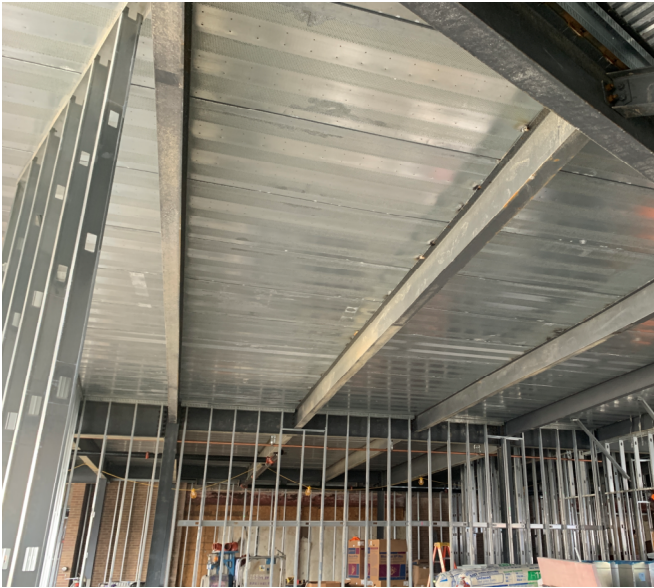
Zone C—Level 1—Interior Framing In Progress
