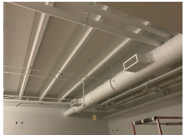
Zone G—Renovation—Permanent Ductwork and Direct Applied Ceiling
