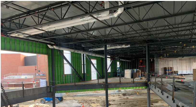
Zone C—Level 2—Addition 2 North
