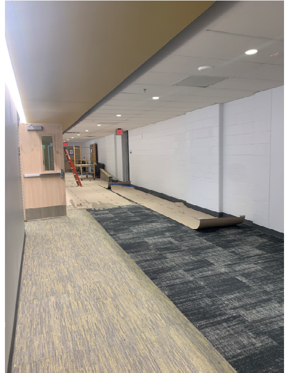
Zone B—Complete Hallway in Level 1
