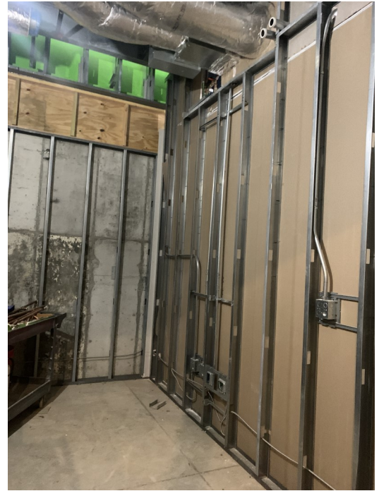
Addition—Level 1 Interior Wall Framing and Drywall
