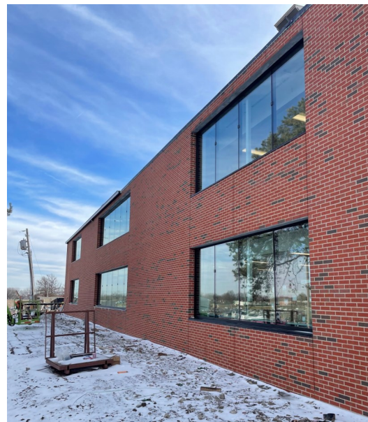
A Building North Face—New Brick Façade and Windows
