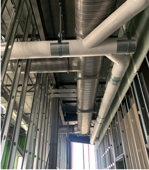
Addition— Level 2—Interior Framing and Mechanical, Electrical, and Plumbing Systems
