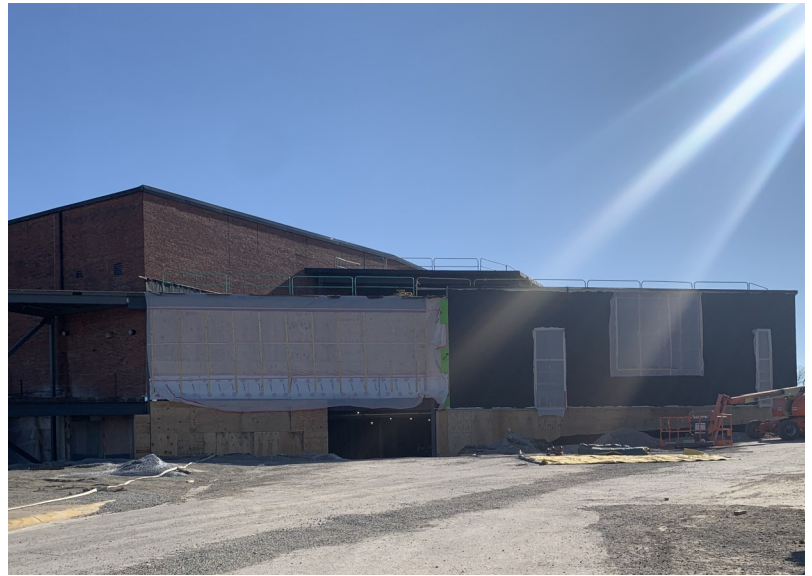
Addition— Exterior Air Barrier and Temporary Enclosures
