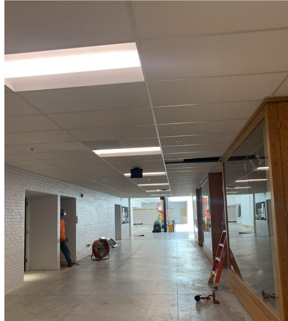
PAC Lobby – New HVAC system, upsized storm drainage, updated ceiling, new LED lights, fresh bright paint
