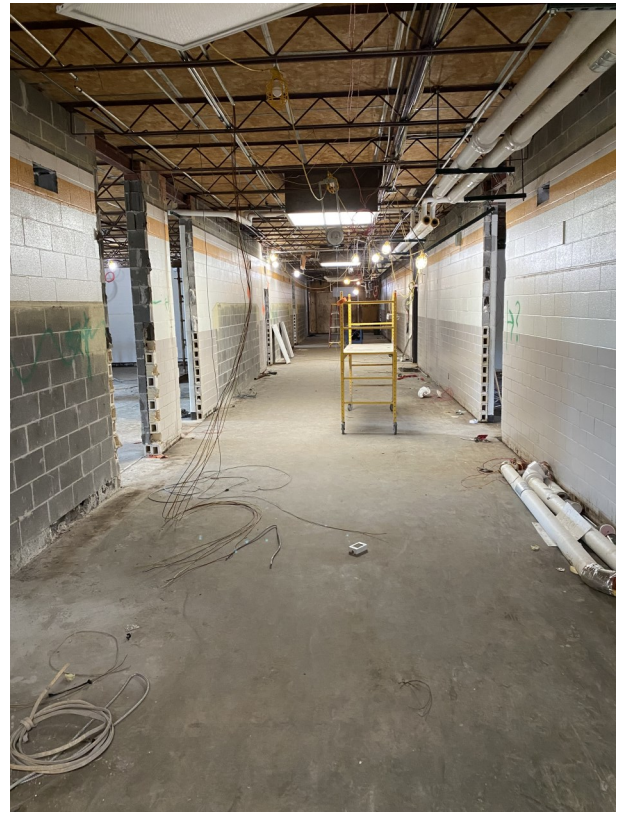
Area B East—Demolition
