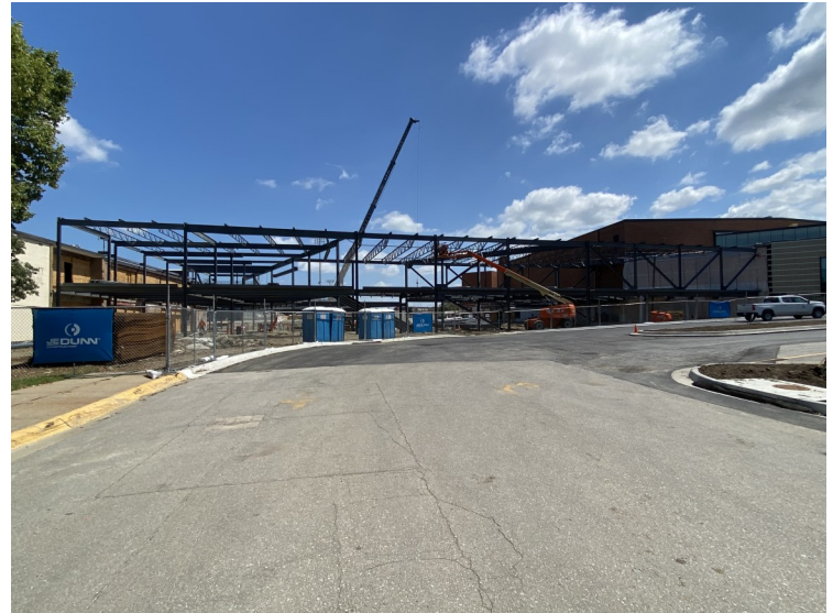
Area C - Addition 2 Steel Erection
