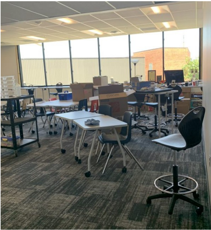
A Building—New Window, Carpet, Ceiling, Lights
