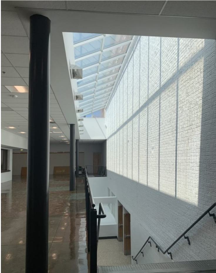
Corridor and Stair Outside Lecture Hall—Updated paint, ceiling, lights
