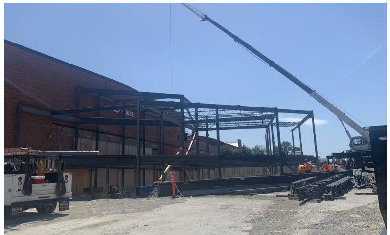
Addition—Steel Erection
