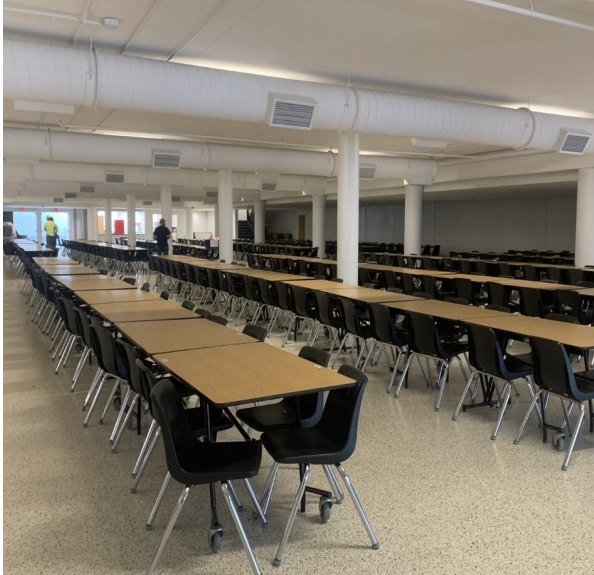
Cafeteria—Updated Ductwork and Paint
