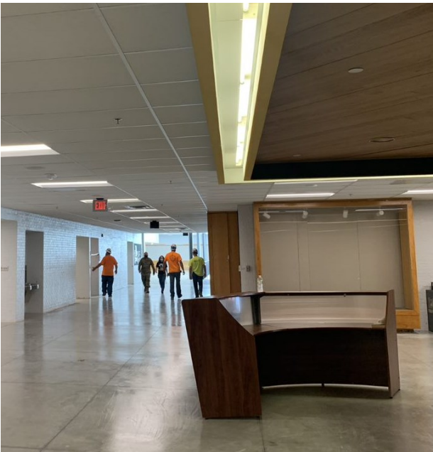
PAC Lobby—New ceiling and lights
