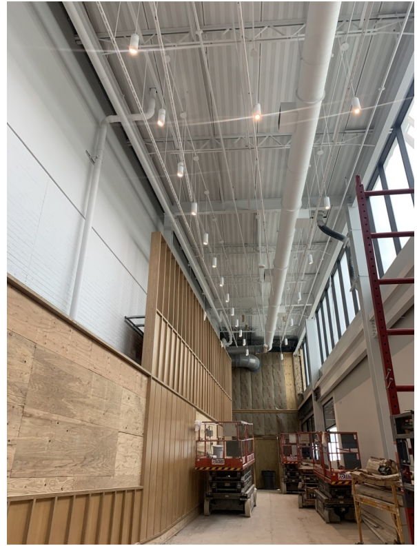
Addition—Level 2 - Wood Wall Installation in Progress
