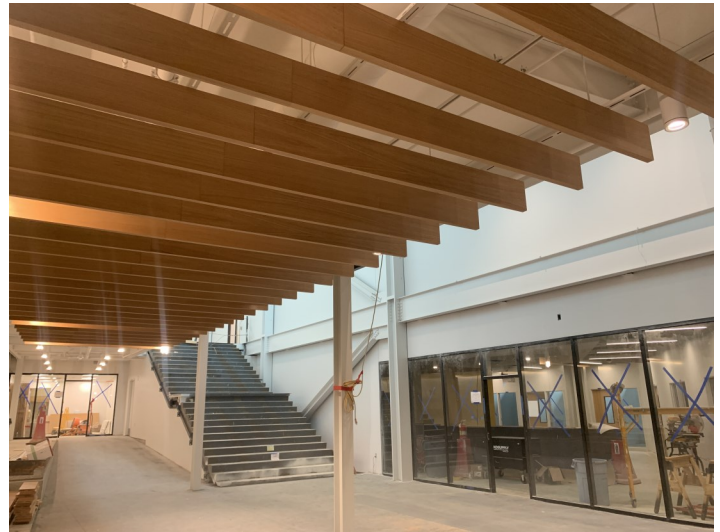
Addition— Wood Baffles in Entry Way
