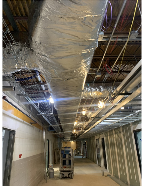
B Level 1 West—Hallway Overhead Work in Ceiling
