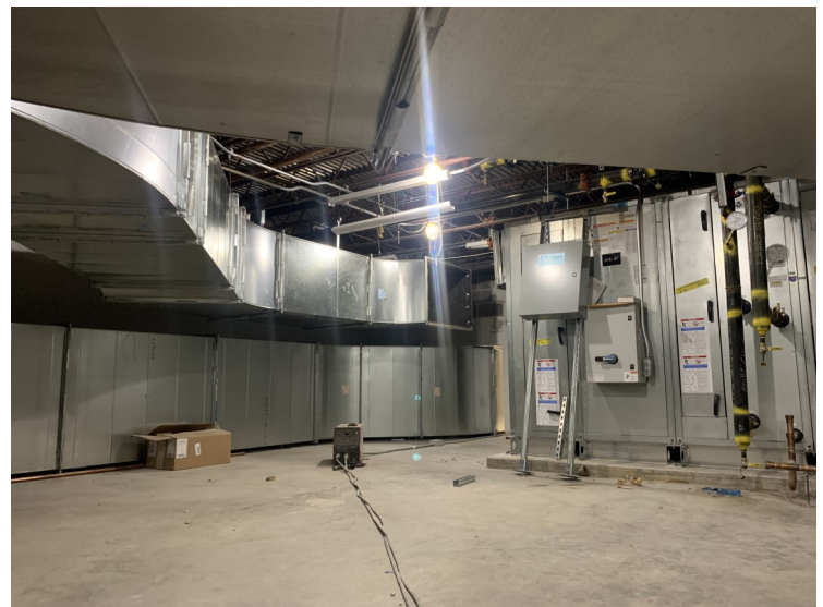
B Basement—New Mechanical Unit and Ductwork
